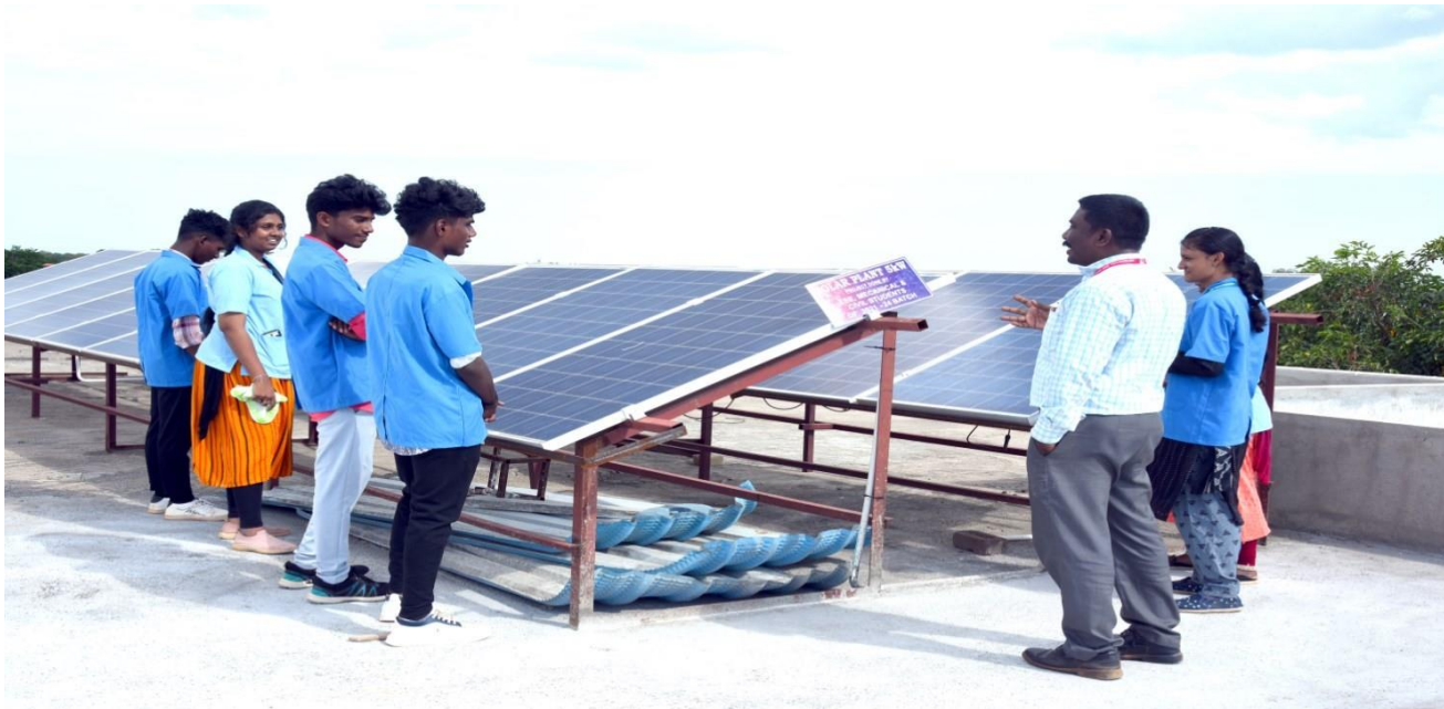
5KW Solar Plant on 2023-2024
